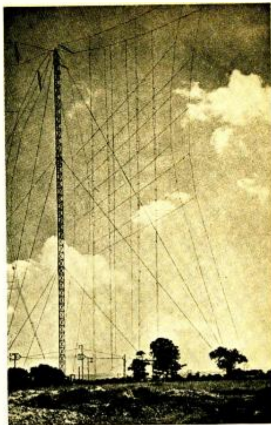
THE AERIAL ARRAY AT DAVENTRY, USED FOR TRANSMISSIONS TO THE FALKLAND ISLANDS AND SOUTH AMERICA, AND, IN THE REVERSE DIRECTION, TO NEW ZEALAND AND THE FAR EAST. (By courtesy BBC)
