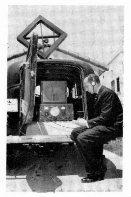
F.C.C. "Police Patrol" equipped with Hallicrafters SX-17 Super Skyrider. Several of these scout cars are in daily use, trapping "bootleggers" and checking other transmissions. Recordings of broadcast programs are also made and sent to Washington for checking purposes.
