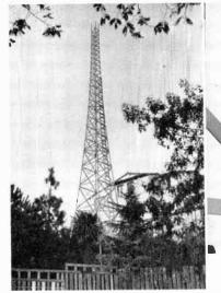
W6QBU's tower, complete except for rotary beam mechanism. Note ladder on right side. Close-up of butt-joint taken from inside of tower and showing how the 2½-in. section joins the 2-in. member.
