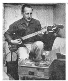
Making a multi-guitar recording with a Series 6 Tandberg tape recorder.
