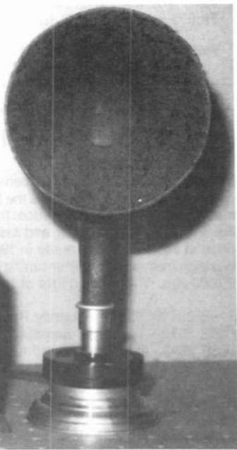
**CLAPP-EASTHAM** - The "Baby Emerson" was manufactured by the Clapp-Eastham Co., Brooklyn, New York. It is a one-tube set using an "Emerson" multivalue type of tube (tube box shown left of set). The small horn speaker shown to the right of radio is of unknown manufacture. (R.A. Hostler - Findlay, OH)
