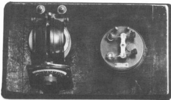
Figure 1. Atwater Kent Crystal Set with Variometer.
