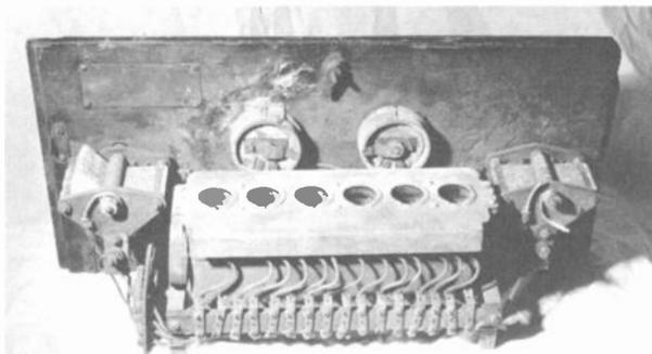
Figure 1. RCA Superheterodyne catacomb assembly from the Model AR-812 Superhet.
