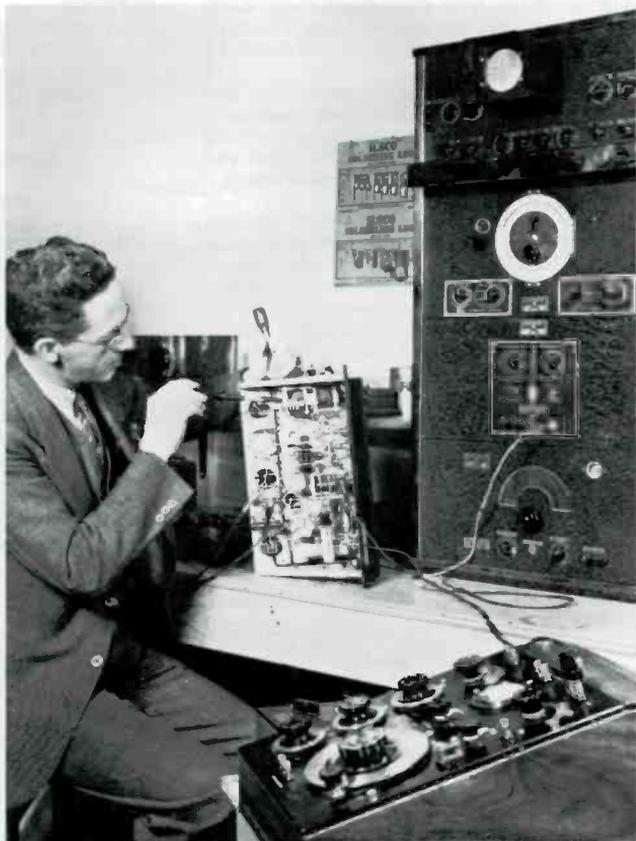
Figure 3. Vintage photograph of a typical setup using the General Radio Type 650-A Impedance Bridge. (Photo courtesy of Ron Boucher.)
