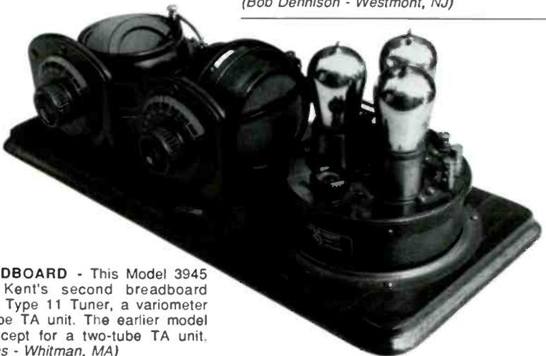
**EARLY BREADBOARD** - This Model 3945 was Atwater Kent's second breadboard consisting of a Type 11 Tuner, a variometer and a three-tube TA unit. The earlier model was similar except for a two-tube TA unit. *(Augie Walackas - Whitman, MA)*
