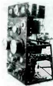
**FOR SALE/TRADE:** WWI 1/2 KW submarine Type C-296-B spark transmitter converted to tube operation in 1938, sold by Mackay Radio & Telegraph Co. manufactured by Federal Telegraph Co. of Newark, N.J. Photos and details available on request. Call today. Scott Shanks, 23707 SW Mtn. Creek Rd., Sherwood, OR 97140
