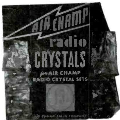
**CRYSTAL DISPLAY** - Air Champ radio crystal elements were sold in packets stapled to this cardboard display. The crystals are mounted in lead within a metal holder. There are fifteen original packets remaining on the board. One corner of the display is broken away. (*Michael Crain - Harveys Lake, PA*)
