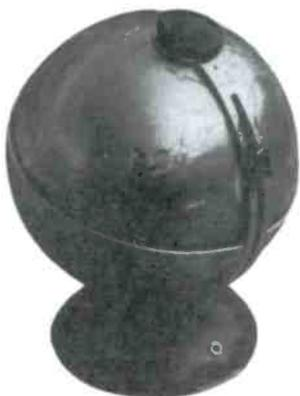
**NOVELTY TRANSISTOR RADIO** - This is the Fleetwood Model NTR-6G manufactured in the early 1960s. It is a transistorized globe radio with a polar ON/OFF/VOL control switch. (John S. Neuman - San Marcos, CA)
