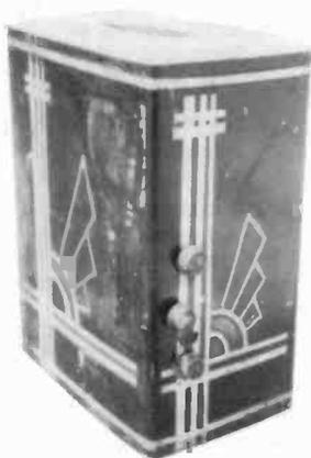
**RCA MODEL R-28-BW** - This 1932 style radio is 20 1/2" high by 8" by 12". The sides are covered with a one-piece tin plate which is fitted flush under the wood top. A Deco design is stenciled on all sides in black. The top, which holds the speaker, is painted silver. The back cover, missing on this one, was apparently also tin plate. It has standard RCA wood knobs and a small dial opening. (Steve Lange - Milwaukee, WI)
