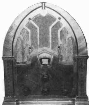
**CROSLLEY MODEL 168** - This 1933 cathedral radio is a seven-tube dual band superheterodyne. The intermediate frequency is 181.5 Kc. (Lyle Scheid - Iroquois, SD)
