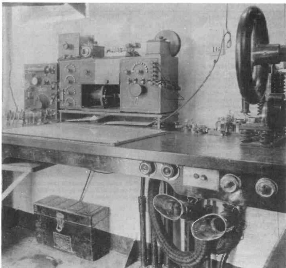
Figure 2. The I-P-76, 1914 model, installed on the U. S. S. Cheyenne. To the left is a De Forest Ultraudion (heterodyne oscillator for CW reception).
