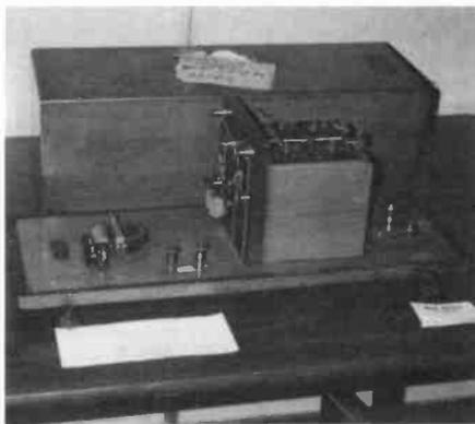
Another contest entry — this pre-1910 German coherer made by Kohl. Note the box with batteries to the right of the detector.
