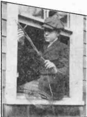
Then the antenna wire is stretched over to the roof of the garage. A long span, high above the ground, brings great results.
