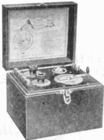
Figure 1. This Aeriola Sr. radio receiving set was a prize to any boy selling over 800 more copies of "The Home Journal" than he had sold in August. The booklet describes the set as "...an up-to-the-minute, reliable 'bulb' radio receiving set. The set is portable and the upkeep expense very small. Outfit includes 1 aëriotron W.D.-11 D vacuum tube, 1 filament dry cell, 1 plate dry battery, head telephone receivers, antenna equipment and full instructions."
