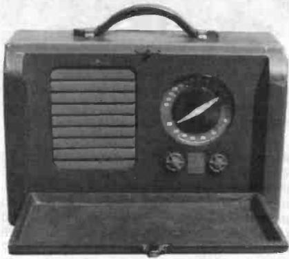
**EMERSON MODEL FU-428** - Made in 1942, this AC-DC battery portable uses a Type 117P7 dual purpose tube — one half for rectification on AC power, and the other half for the output on AC-DC power. On battery power it uses a 3Q5 output tube. (Doug Burskey - Mansfield, OH)
