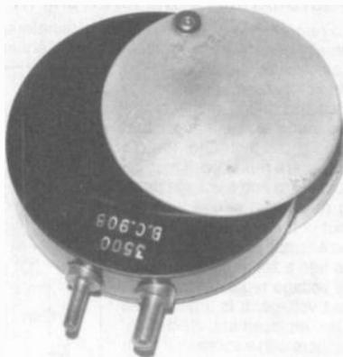
Figure 3. GECophone loading coil with adjustable aluminum vanes. Three different ranges were available; this one was designed for 1200-1850 meters for reception of the Paris Radiola station.
