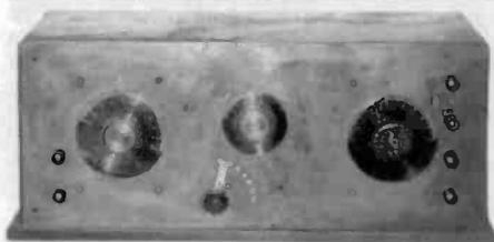
**HOME BREW BATTERY SET** - This homemade tuner, probably made before 1920, used 2 wooden variometers with solid wood rotors and a tapped variocoupler wound on an Armour and Co. oatmeal box. The dials look like celluloid and consist of 2 pieces that can be removed by unscrewing a binding post nut in the center. (*George Hausske - Wheaton, IL*)
