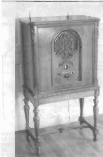
**SPARTON MODEL 610** – A TRF design of simple yet sturdy construction, this set has 5 stages of RF amplification giving good performance on weak signals. Three separate chassis house the tuning condenser, RF stages and power amplifier. (Greg Jones – Westerly, RI)
