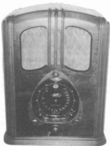
**ZENITH MODEL 9-S-232** – Now also known as a "Walton" radio, this ca. 1937 set is the export version employing 9 tubes. It does not have the motorized tuner but does have a selectable operating voltage and a phono input on the rear of the chassis. (*Herb Parsons – Peabody, MA*)
