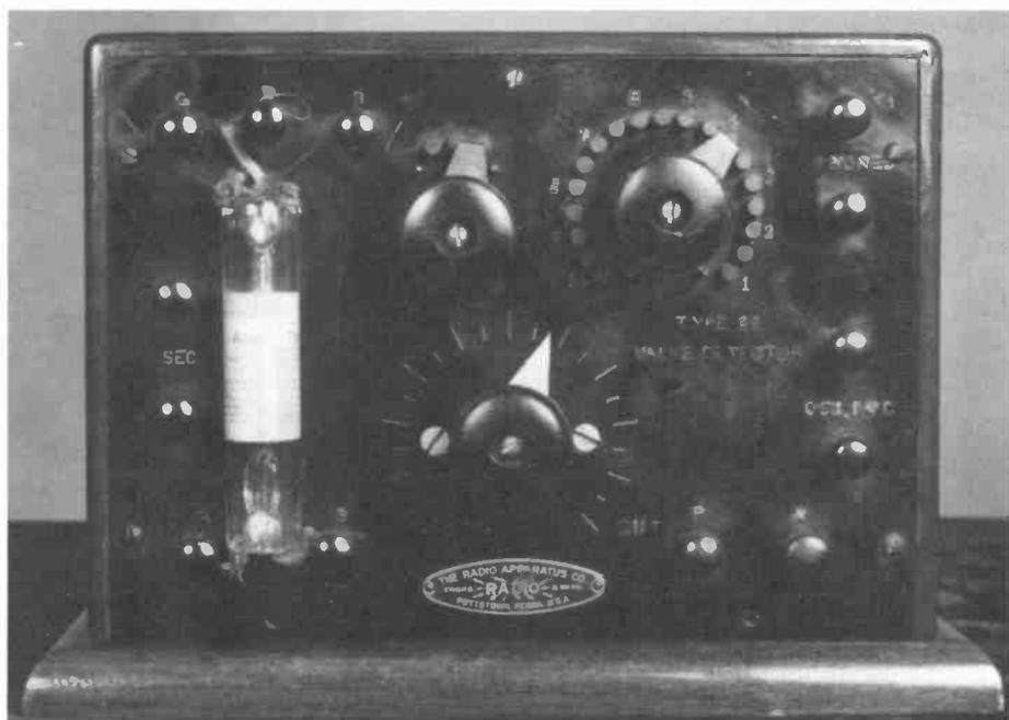
Figure 6. Panel view of the Type 36 valve detector. The tubular audion shown is a vintage replacement and not the Liberty valve furnished by the Radio Apparatus Company.
