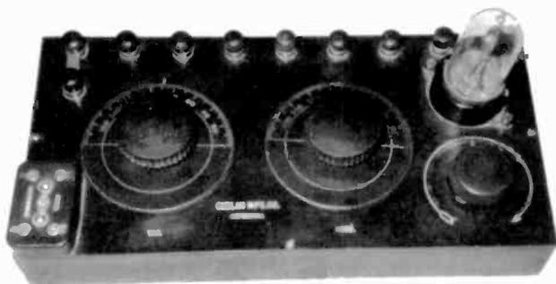
**GIBLIN MANUFACTURING CO. MODEL UNKNOWN** – Made in the early 1920s, this 1-tube set measures 5½" x 11" x 1½". Giblin of Pawtucket, R. I., is better known for its "Radioear" crystal set. (Ed Bell – Raleigh, NC)
