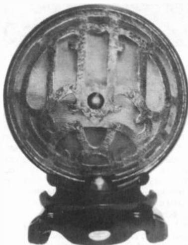
**BORKMAN RADIO CORP. MODEL 18** – Also known as “The Chinese Cone-Flex,” this unusual speaker resembles a cone-type speaker, but consists of a papier-mâché facing the side. The driver is located in the base. The speaker is 19" high. (*Ed Bell – Raleigh, NC*)
