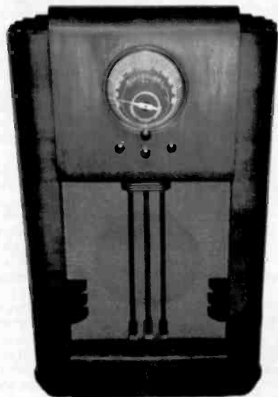
WILCOX-GAY MODEL 6T11 — This 11-tube console with tuning eye has a unique white-on-black glass dial marked for broadcast, police and foreign bands. It features dual Type 80 rectifier tubes with Type 6F6 push-pull output. (Ronald L. Gamer — Excelsior, MN)
