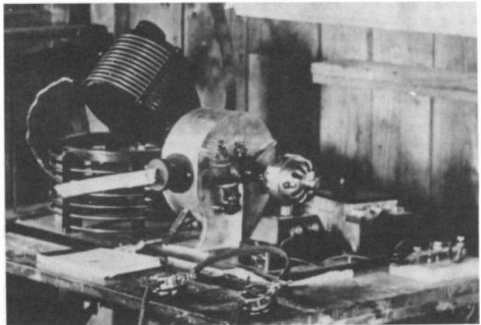
*Figure 2. The World War I era wireless transmitter, an enlarged view from the cover of this issue.*
