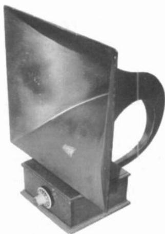
**CALLOPHONE HORN SPEAKER** – The huge metal horn bell on this speaker measures 15" square. The driver inside the rear of the wooden box is adjusted for tone by the front dial which has a long shaft to the driver. Manufactured by the Callophone Co. of New York City, it sold for \$35 in 1924. (*Dave Crocker – Mashpee, MA*)
