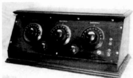
Figure 3. A front view of the 5-tube Chelsea Super-Five, manufactured in 1925.
