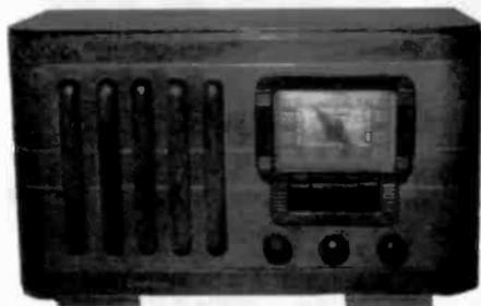
**TROUBADOR, MODEL UNKNOWN** – This 6-tube AM band radio, ca. 1947, was made by Warwick Manufacturing Company. It features the "Troubascope Looptenna." *(John Phipps – St. Charles, MO)*
