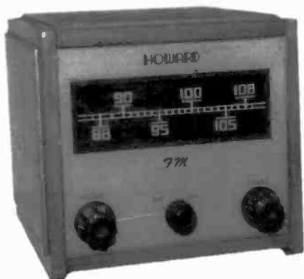
**HOWARD MODEL 482** – This is an FM converter manufactured by Howard Radio of Chicago. It is used to tune an AM radio to FM by plugging into the phono input terminal. (*John Phipps – St. Charles, MO*)
