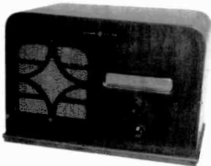
**GENERAL ELECTRIC MODEL U50** – This battery-operated farm radio uses the following tubes: Types 30, 32, 1F4, 34, 1A6. (*Clark Trissell – Lincoln, NB*)
