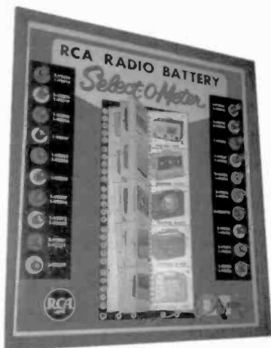
**RCA "SELECT-O-METER"** – This RCA battery selector for portables would be found at a repair counter for public use. First, one would locate the radio of interest from the spiral-bound center pamphlet, and then, using the wire, plug into the jack indicated. One of the lights on either side would then indicate what battery combination was required. A "D" battery, placed in the space at lower right, powered it all. (Paul Check – Lodi, NJ)
