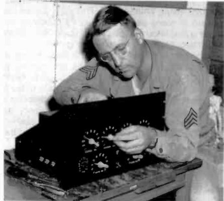
*Figure 2. In this photograph, then Sergeant Scribner is shown putting the finishing touches on an amplifier that he built for use in the Post Broadcasting System.*
