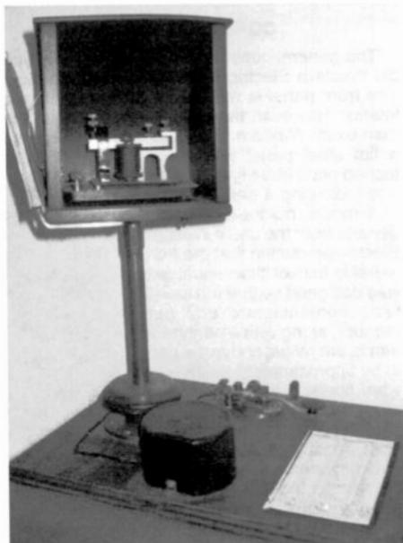
Figure 2. Telegraph sounder and resonator.
