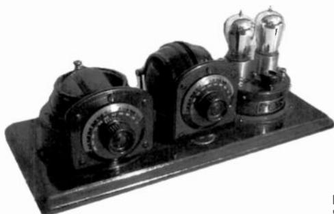
**ATWATER KENT TYPE 3925** – This 1925 breadboard receiver is sometimes called the Model 1, for it was the first of this type of Atwater Kent board receivers. On the left is a coupled circuit tuner; in the middle, (installed only by the local dealer), is a variometer to make it regenerative; at right is a 2-tube TA unit, all mounted on a mahogany board. This set sold for \$32, without the variometer, and \$42 complete, without tubes. (*Dave Crocker – Mashpee, MA*)
