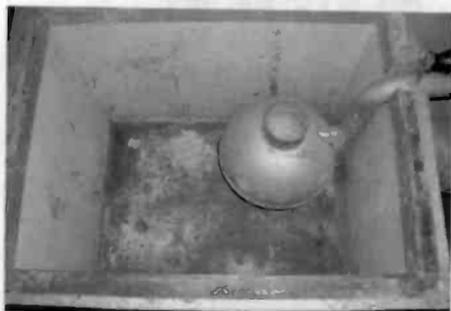
Figure 4. The cold ball portion of the refrigeration unit is shown placed in the Icyball's insulated cabinet.
