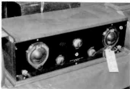
A Smith & Nordstrom 5-tube TRF battery set in a wooden cabinet with an inlaid top cover. The set uses an unusual triple-gang tuning capacitor.
