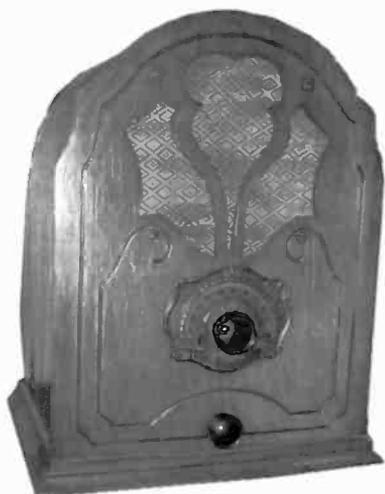
**CRC RADIO CO. "KING"** – The only clues to the identity of this small cathedral are the word "King" on the dial escutcheon and "CRC Radio Co., Chicago, Illinois" on the chassis. About 13 inches tall, it is a 4-tube, transformer-operated TRF, using two Type 24A tubes, one Type 47, and one Type 80. If you recognize it, please send details to A.R.C. (Tom Ackerman – Germantown, IL)
