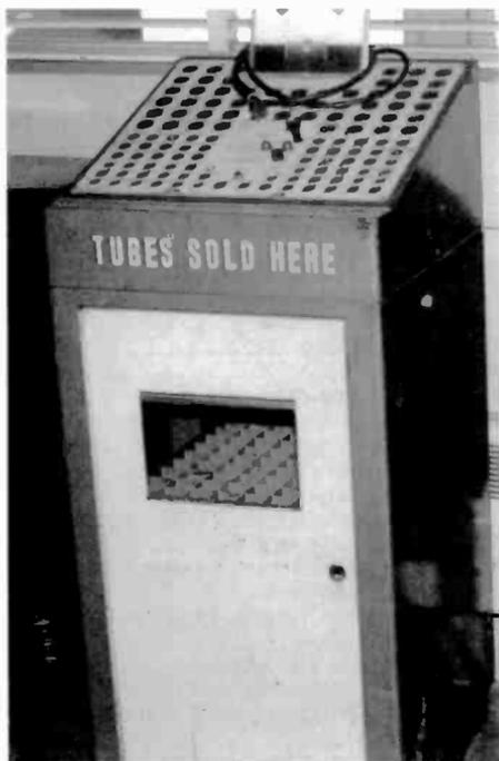
This typical "drugstore" type tube tester uses multiple tube sockets to simplify testing. It sold for \$60.
