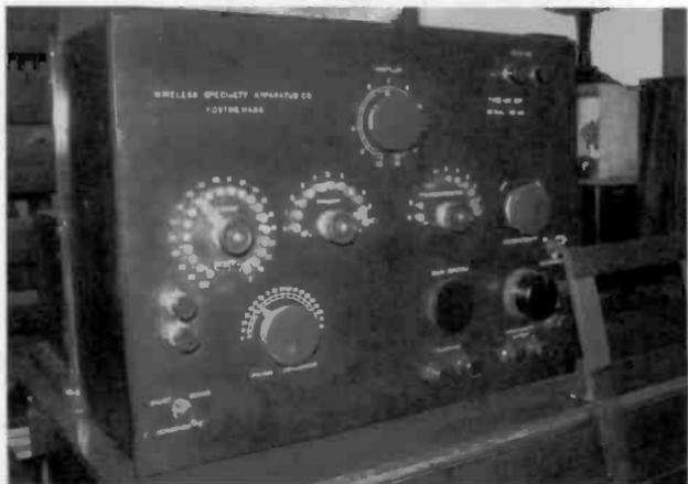
Figure 9. Panel view of the Wireless Specialty Apparatus CR 1917.
