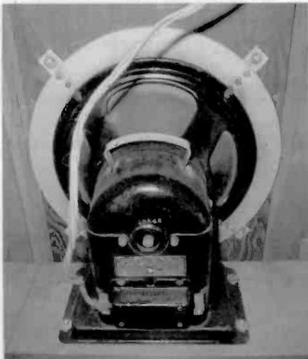
Figure 2. The large and heavy speaker for the Fada 290C.
