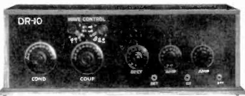
*The DR-5 and DR-10 Busco receiving sets. The DR-5 is "built for the enthusiast who desires a modern compact and efficient receiver for broadcast reception." The DR-10 "has been designed and built expressly for concert reception." The DR-5 uses a single tube as detector. The DR-10 adds a two-stage amplifier.*
