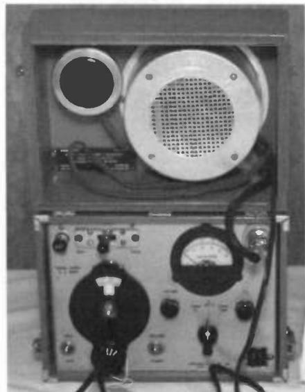
Used in isolated lookout towers, this Forest Service 2-way radio, Model SPF, from the 1930s, operated on 3.2 MHz. In a carrying bag with batteries, it weighed 20 pounds.
