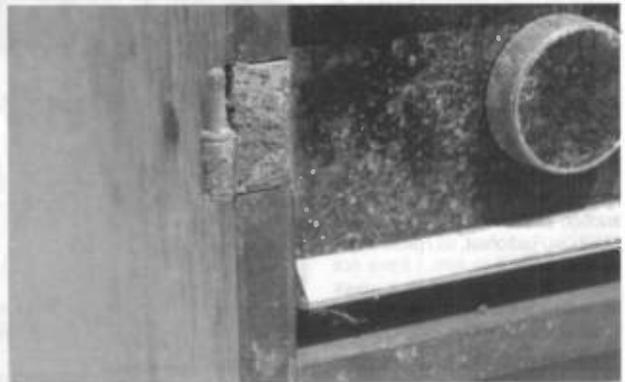
Figure 4. An example of damage to the wood, hinges, panel, and knobs can be seen here.
