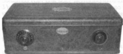
**ATWATER KENT MODEL 38** – Atwater Kent Mfg. Co. of Philadelphia manufactured this 8-tube receiver in 1927. It is housed in a wrinkle-finished metal box and was the last of this series to display the famous gold design on the lid. (*Clark Trissell – Lincoln, NE*)
