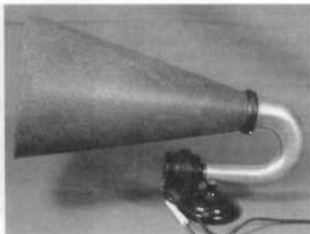
Made by Murdock, this odd horn speaker with a fiber, megaphone-like horn sold for \$325.
