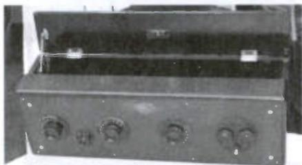
*The Model 5A is similar to the Model 20, but the orientation of the RF coils is different. The tag says "Type 5A" and there is no serial number.*
