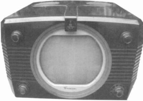
**Emerson Model 614** - This television was manufactured in 1950. The cabinet is made of bakelite and the chassis uses a 10" CRT. Very stylish but must weigh about 40 pounds. (*William Franken - Bogata, NJ*)
