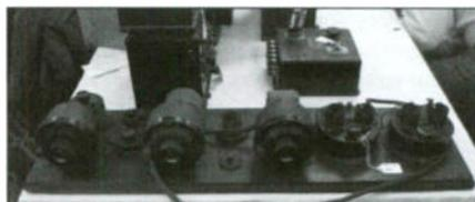
An Atwater Kent breadboard battery set.
