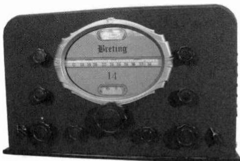
**Breting model 14** – Manufactured in 1937. The frequency coverage is from 550 kc to 34 mc. It has 14 tubes and originally sold for \$100. Rudy Gertz, Omaha, NE
