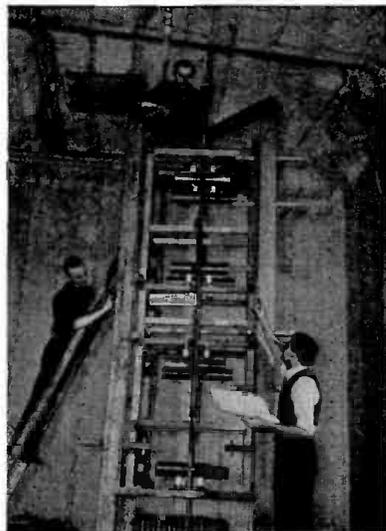
(Above) TELEVISION ANTENNA developed by the General Electric Co. at Schenectady for use with its studio-to-station transmitter. Main transmitting station is located in the Helderberg Mountains, 12 miles away. Isolantite insulators of stand-off and lead-in variety and radio transmission line equipment are extensively used in connection with special television apparatus — as in other phases of the radio and communications industries.
