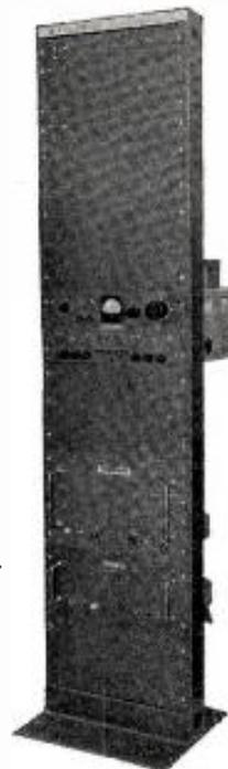
▶ **Transmitter**—The Philco Model TLR-6 Transmitter consists of three basic units: (1) a transmitter chassis, (2) a +750 volt dc power supply and (3) a +300 volt dc power supply. All units are designed for rack mounting in a standard 19" relay rack.
