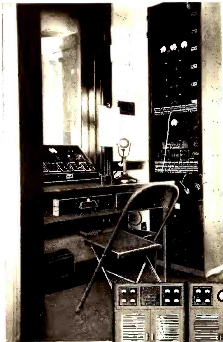
Part of control room at KSD, where RCA Speech Input equipment is used throughout.
