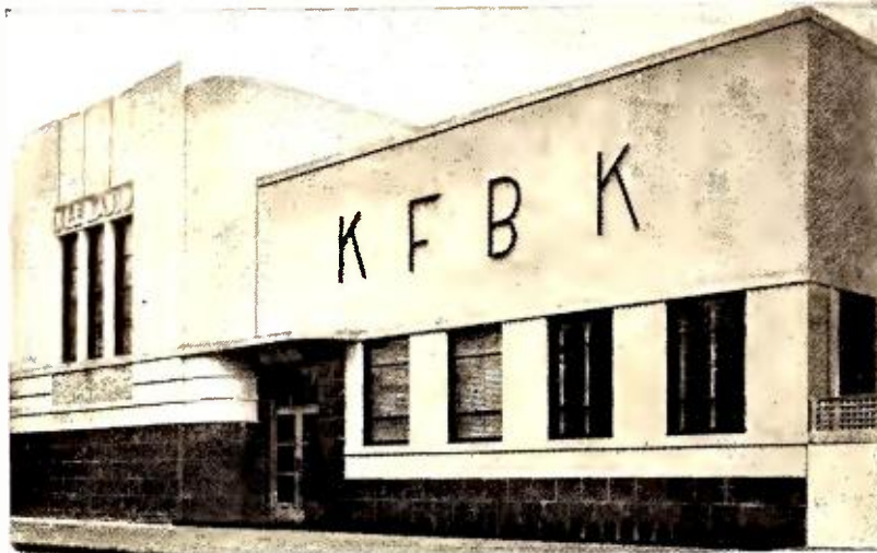
UTILITY AND BEAUTY—Modernism combines with practicality in the new studio building of KFBK, Sacramento, Cal., dedicated last month on the occasion of the station's rise to 5,000 watts on the new 1490 kc. frequency. Harry J. Devine, of Sacramento, was the architect; Robert L. Cramer Co., San Francisco, the acoustic engineers; Frank Maloney Co., general contractors in the modernization project.
