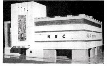
ARCHITECT'S scale model of the much-heralded NBC building in San Francisco showing the building costing over a million dollars which will house studios and technical equipment for KGO and KPO. Five stories high, it is constructed of reinforced concrete, trimmed with bands cf translucent glass brick. There are no windows, the structure being air conditioned throughout. The building will provide 52,800 square feet of floor space, more than double the present quarters.
